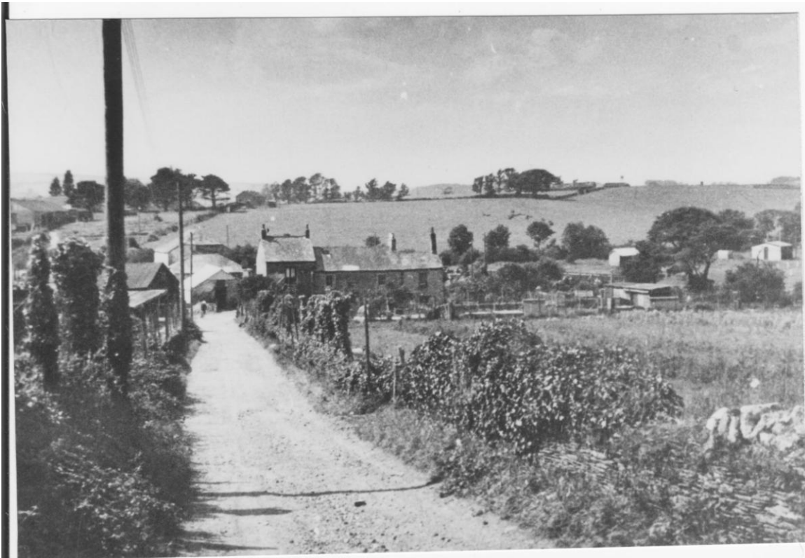
Lane to Mill and Farm
