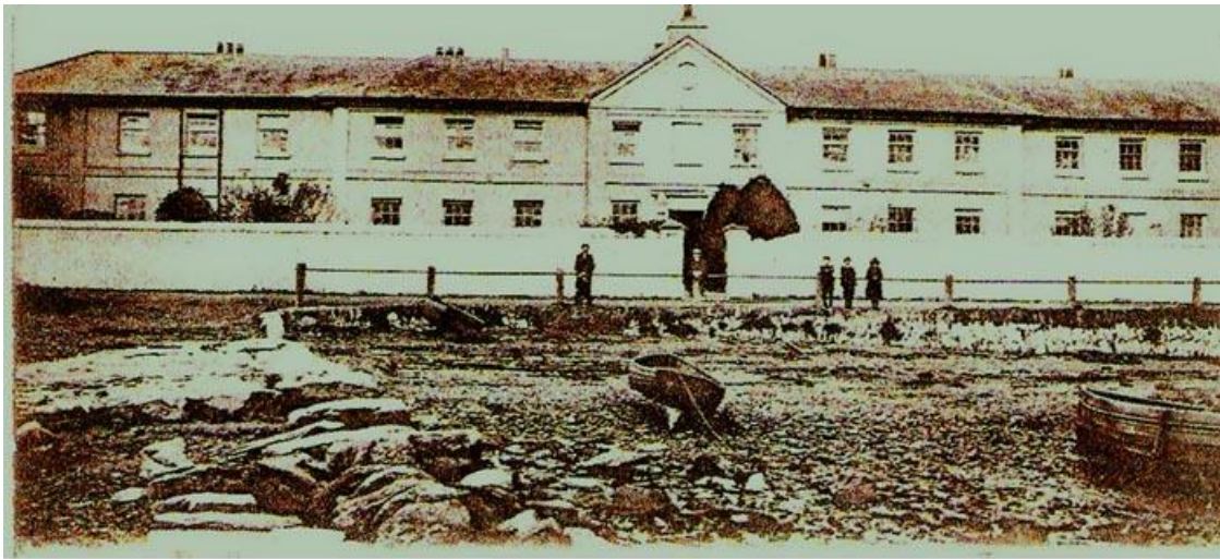
The Union Workhouse, Union Road built 1839.
