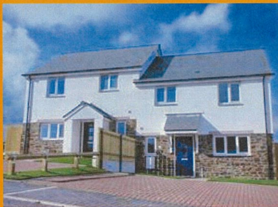
Rame (Wendron), Cornwall CLT and Coastline Housing, 16 Affordable Homes
