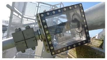
The photo above shows the preliminary cable clamps and a weatherproof enclosure with cable monitoring equipment already installed, and the graphic below illustrates the planned remedial work. This work is currently expected to be completed in June 2023.
