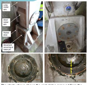
The photo above shows the end plates removed from the rocker pin with visible wear allowing unwanted vertical movement of the rocker arm.
