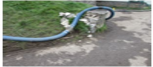
Retaining wall next to Pumping Station Chapeldown Road
