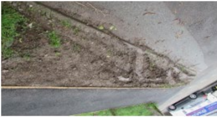
Junction of Carbeile Road/Chapeldown Road
