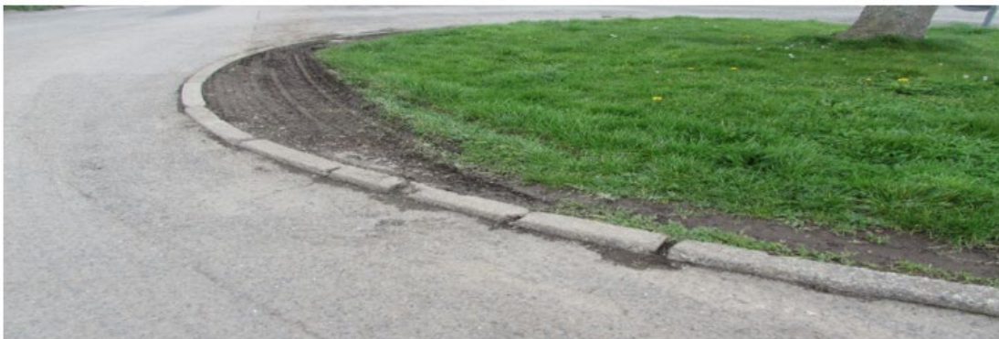
Roundabout junction of Sango Road and Chapeldown Road
