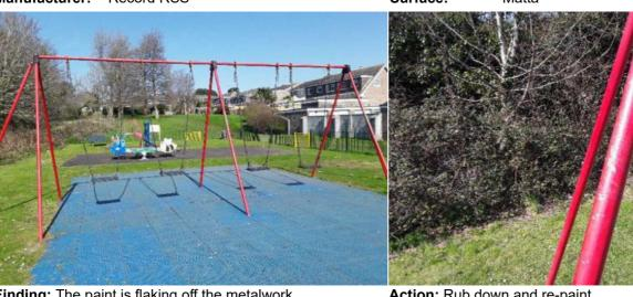
Finding: The paint is flaking off the metalwork
