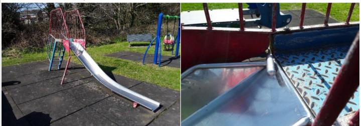
**Finding:** There is/are finger entrapment/s in the frame and Action: Monitor - No remedial work recommended the item fails to meet the requirements of BS EN 1176 Part 1 4.2.7.6 Entrapment of fingers
