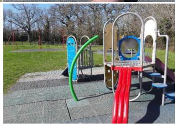
**Finding:** The green firemans pole has been installed too far **Action:** Monitor, no remedial action is recommended away from the structure in contravention of the manufacturers specifications
