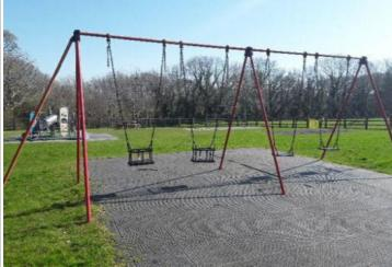
**Finding:** The surfacing mats have separated, are not secured and can be lifted creating trip points. The gaps between the mats are also large enough for a small foot to enter
