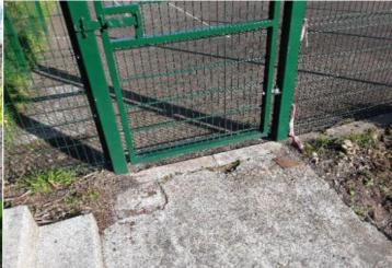
**Finding:** There is moderate damage to the concrete surface **Action:** Repair the damaged areas of surfacing near a gate
