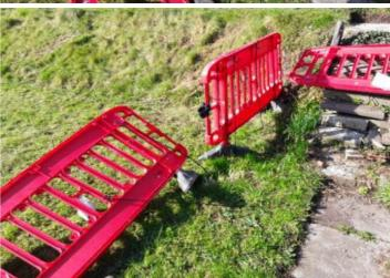
**Finding:** The steps on site has been isolated from use however the area is still accessible and the means of isolation has either introduced additional hazards that may cause harm in the event of users accessing the area or is insufficient to stop users from accessing the steps
