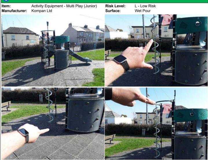
**Finding:** There is excessive movement in the corkscrew due to loose or missing fixings
