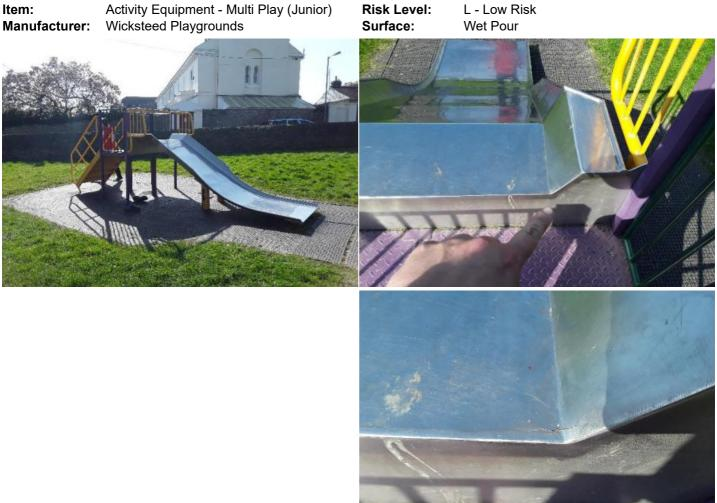
**Finding:** There are fractures or cracks in the slide start section
