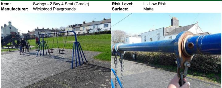
Finding: The Anti Wrap bearings are dry and not moving freely
