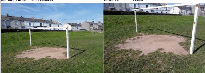
Finding: The surface has eroded in some areas
