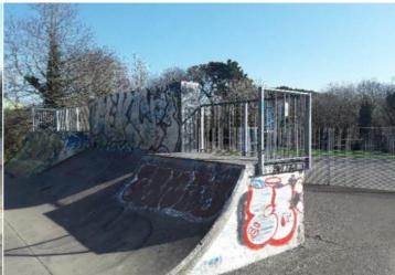
**Finding:** Barrier ends should have a radius of at least 50mm **Action:** Monitor, no remedial action is recommended as required by BS EN 14974
