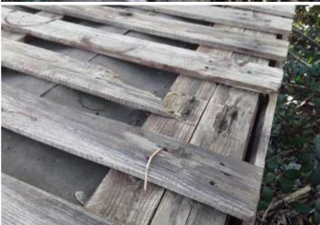
**Finding:** There are areas or parts of the timber on the structure that have rotted
