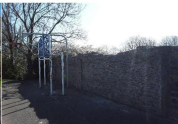
**Action:** Repair as required to remove / secure all loose rocks, remove debris from the surface and maintain
