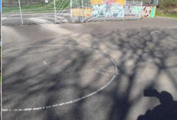
Finding: The bitumen surface is worn or damaged
