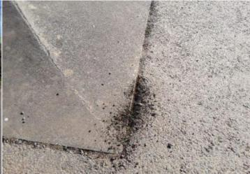
**Finding:** Joints between the riding surfaces should not be **Action:** Take corrective action to ensure that the gaps greater than 5mm to meet the requirements of BS EN 14974 between the joints do not exceed 5mm
