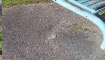
**Finding:** There is some evidence of fire damage to the surfacing
