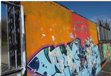
Finding: The paint is flaking off the wall
