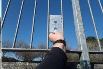
**Finding:** The horizontal opening in the barrier is in excess of **Action:** Monitor - No remedial work recommended 89mm and fails the requirements of BS EN 14974
