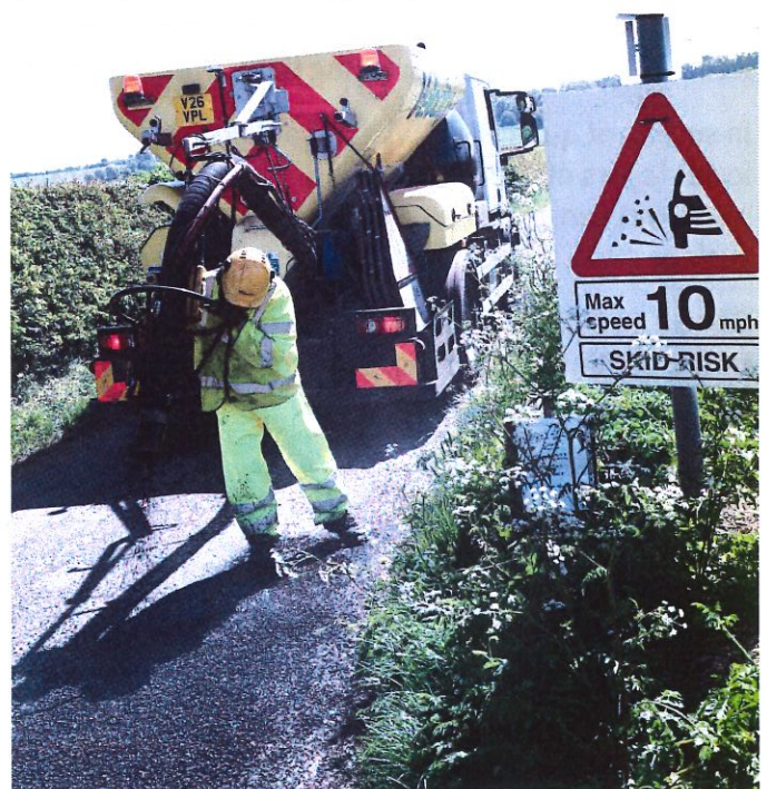
Spray injection machine in use
