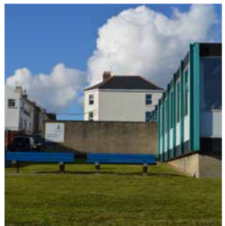
Existing community facilities
